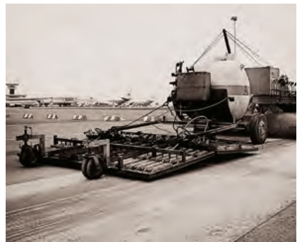
SF 3800 hot milling machine in operation at Düsseldorf Airport in 1973.
