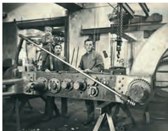
A world premiere in 1932: Hamm's all-wheel-drive tandem roller exhibited superior traction and compaction characteristics. This photo shows the unfinished first prototype.
