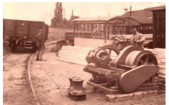
In this photograph from 1925, a transfer table from Vögele at the port of Mannheim connected two parallel train tracks, making it possible to swap locomotives.
