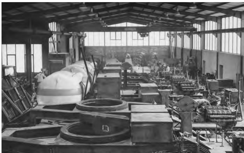
What started as a workshop soon developed into a production hall.
