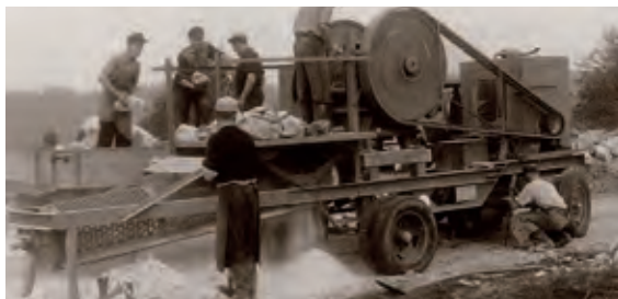
Kleemann developed the first wheeled mobile jaw crushers with drum screens in the 1950s.
