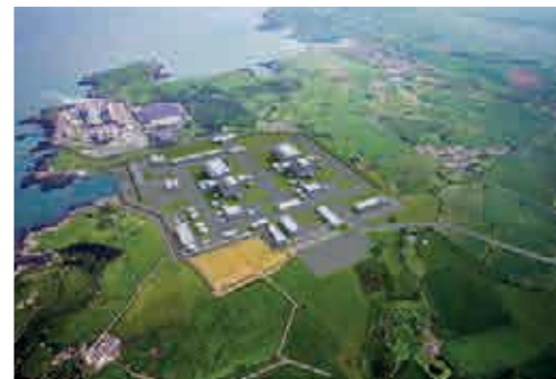
Power systems and equipment
