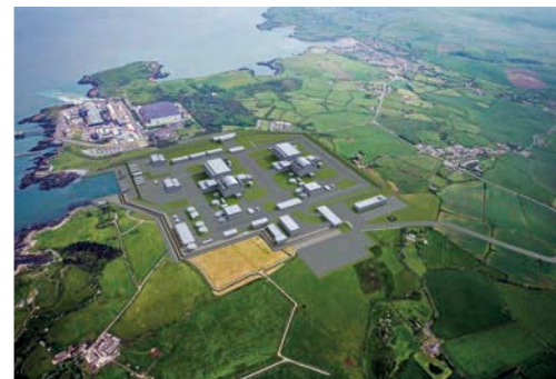
Power systems and equipment
